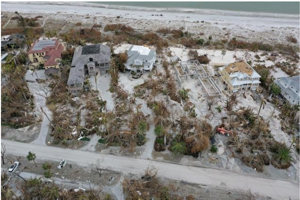
The hurricane damaged nearly every structure on Sanibel, shown here in early October 2022. Though rebuilding efforts will likely last years, some businesses have opened their doors once again. PHOTOGRAPH BY JOE RAEDLE, GETTY IMAGES
